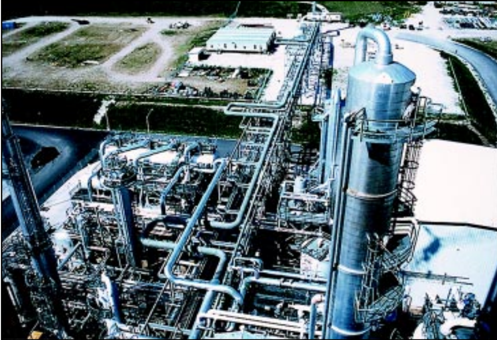
The gas cleanup system removes H 2 S from the fuel gas; sulfur is recovered as a by-product and sold. Ammonia is also removed and recycled to the gasifier.
